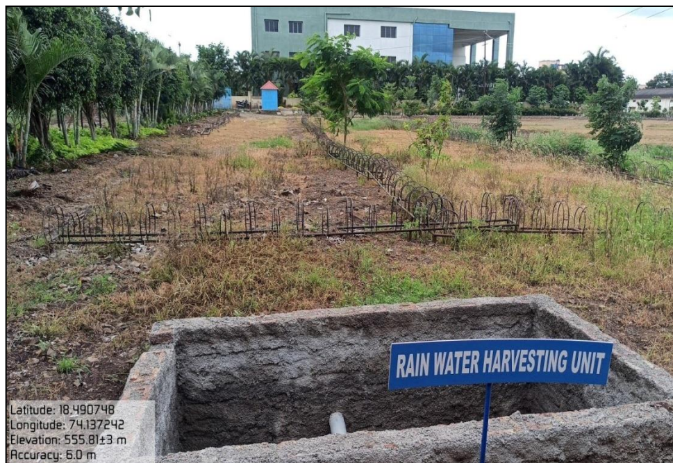
Figure: Rain water harvesting unit
