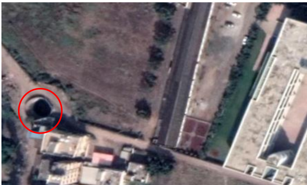
Figure: Main Water Source of PDMC College (locally known as ‘Manibhaichi vihir’)
